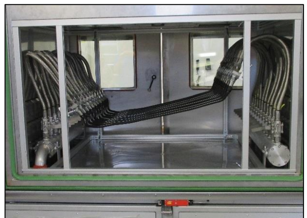
Construction inside the chamber
