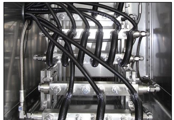
Construction inside the chamber (Depends on chamber)
