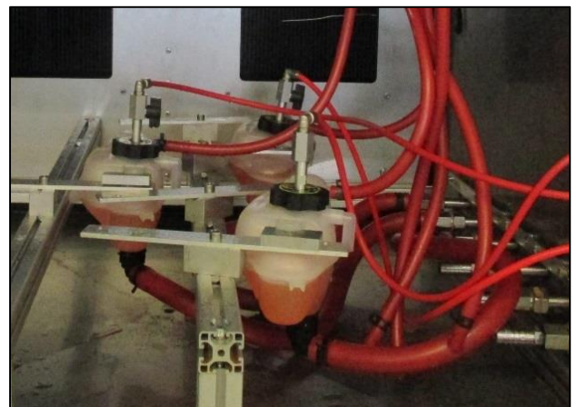
Construction inside the chamber
