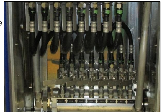
Construction inside the chamber (Depends on chamber)
