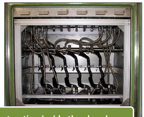
Construction inside the chamber
