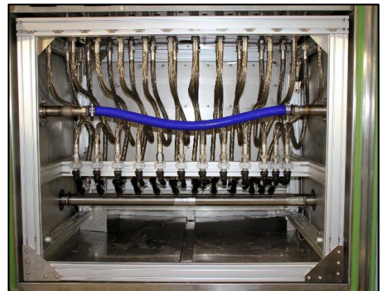
Construction inside the chamber
