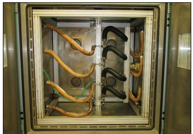
Construction inside the chamber
