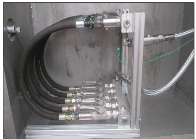
Construction inside the chamber
