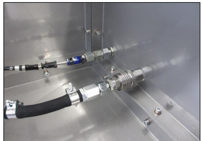
Construction inside the chamber
