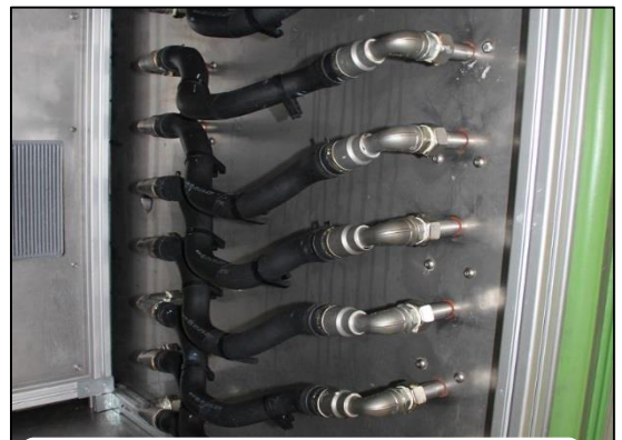
Construction inside the chamber
