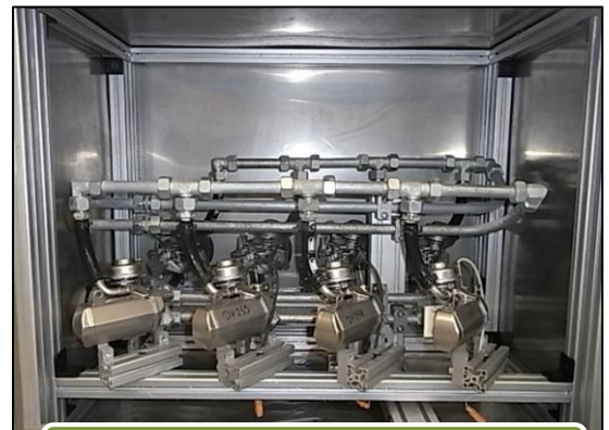
Construction inside the chamber
