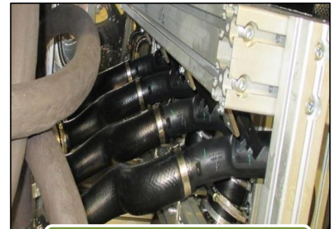
Construction inside the chamber (Depends on chamber)
