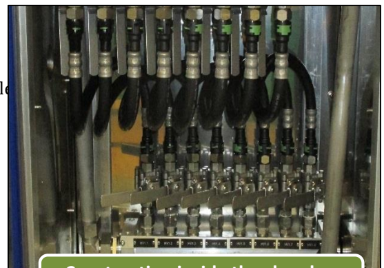
Construction inside the chamber (Depends on chamber)
