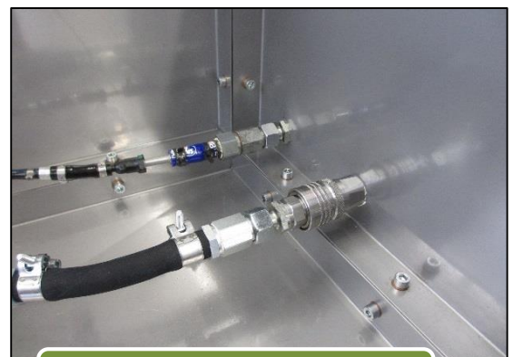
Construction inside the chamber
