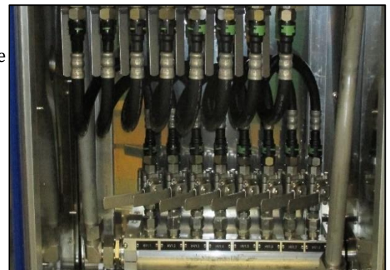
Construction inside the chamber (Depends on chamber)
