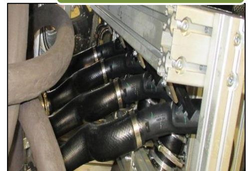
Construction inside the chamber (Depends on chamber)
