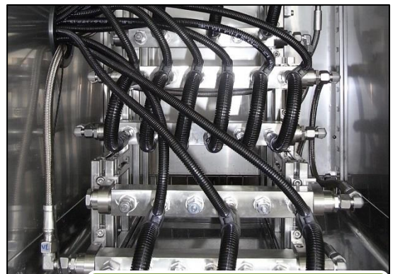
Construction inside the chamber (Depends on chamber)
