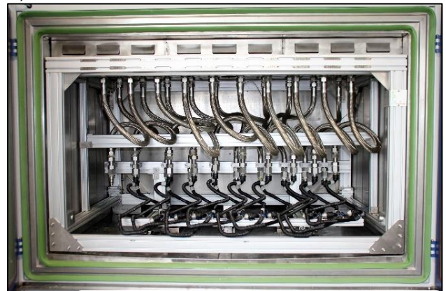
Construction inside the chamber
