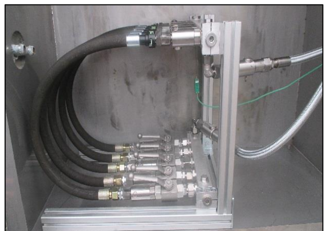
Construction inside the chamber
